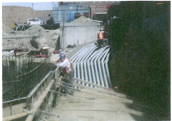
Adams Electric workers ran power conduits from the central plant to the new addition through an underground trench.
