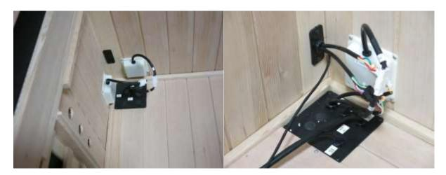
Locate the electrical switch on the black Master Control Box and ensure the switch is on.
