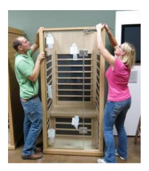
**Note:** Secure the door from falling open and breaking while setting the Front Wall panel. It may be helpful to use your knee to help push in the Front Wall panel while lowering into place.
