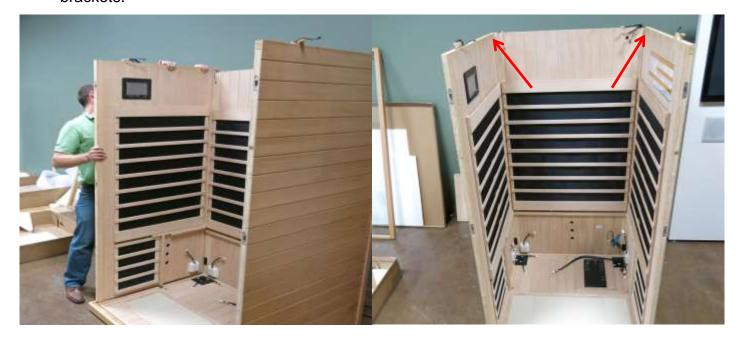
Note: When wall panels are connected in place properly the corners will be flat on top, notice the illustration above right. The right wall is incorrect; the left wall is the correct installation.
