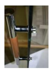
Step 5. Attach exterior portion of door handle on to bolt section and tighten all four set screws with Allen wrench.
