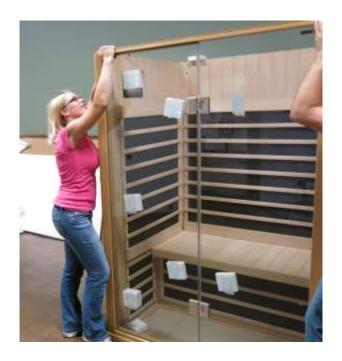
**Note:** Secure the door from falling open and breaking while setting the Front Wall panel. It may be helpful to use your knee to help push in the Front Wall panel while lowering into place.
