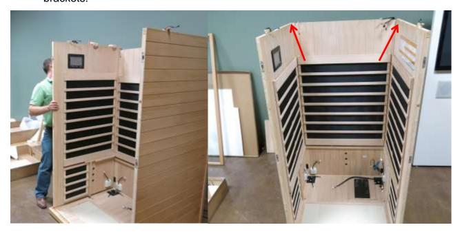
Note: When wall panels are connected in place properly the corners will be flat on top, notice the illustration above right. The right wall is incorrect; the left wall is the correct installation.
