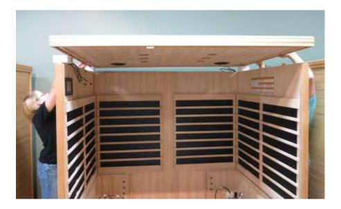
• Once the Ceiling panel is lined up directly above the Wall panels; insert the wires harnesses from the wall panels into the holes in the Ceiling panel.
