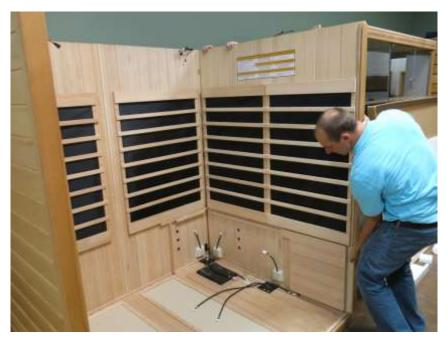
Note: When wall panels are connected in place properly the corners will be flat on top. If one panel sits up higher than another, the panel is not locked in place properly or there is something under the panel.
