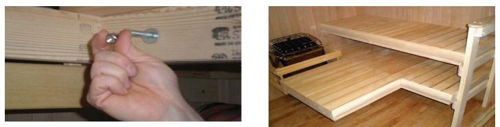
Step 15: Line up the pre drilled hole in the bottom bench with the middle platform bench and attach using lag bolts (provided). Tighten lag bolts to assure rigid bench strength. Repeat this bench installation process on the left side.
