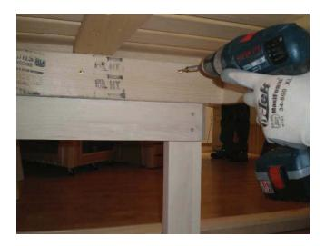
Step 9: Using 2" torx screws (provided), secure the bench to the arm rest assembly. Do this from underneath as shown above.
