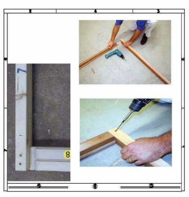
sliding the panels together. To join the tops of the panels together using the provided wood tack jointers.
