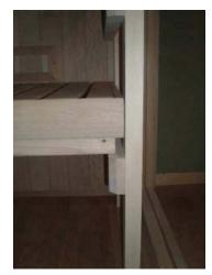
Step 8: Place the lower bench on the backwall support and the lower bench support of the arm rest. Make sure that the decorative bull nose molding is on the front half of the bottom bench.
