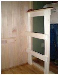
Step 7: Find the free standing (already assembled) arm rest assembly. Make sure that the rounded handle points inward and the ladder supports of the arm rest face inward toward the room.
