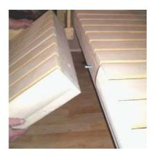
Step 14: Install the middle platform bench making sure that the decorative bullnose is facing the front of the room. Make sure to support the middle bench until connected to the opposite main bench. You may also install the other set of main benches and then install the lower filler bench.
