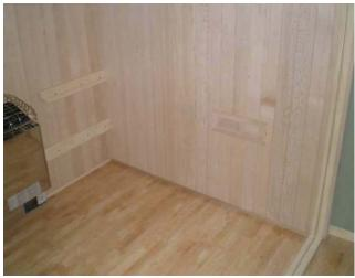
Step 6: Prior to installing the all glass front, start on the right side of the room and note that the bench supports on the back wall have been preinstalled.
