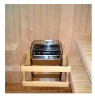
Step 13: Install heater guard around the heater making sure that it is evenly spaced around the heater, (refer to the Heater Instructions for appropriate spacing). The top of the heater guard should be even with the top of the shroud.
