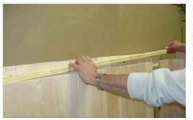
NOTE: After the back & side walls have been set on the base rail, install the top plate using 2" screws. Use 3-screws on each wall.
