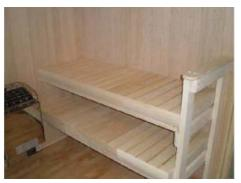
Step 11: Place the top bench on the supports as you did with the bottom bench and secure in a similar manner as the bottom bench. Note the partial bullnose molding on the bottom bench as noted earlier in Step 5.
