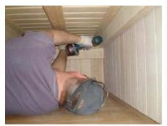
Step 10: Place the top bench on the supports as you did with the back wall. Do this from underneath as shown above.
