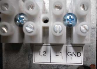
Step 4: "L1", "L2" and "GND" is for the main power feed from the wall outlet. This will be the main power feed for the sauna. Refer to the sauna heater manual for heater specifications.
