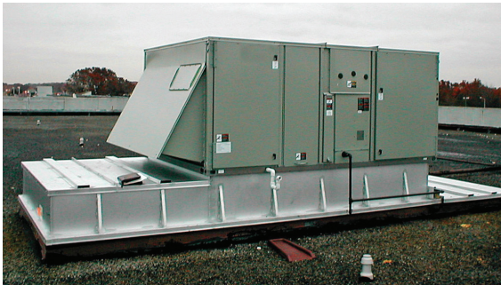
Figure 4: Rooftop HVAC unit in Michigan where a newly installed AEGIS® SGR Bearing Protection Ring reduced shaft currents by 92% to levels well below those that damage bearings.
