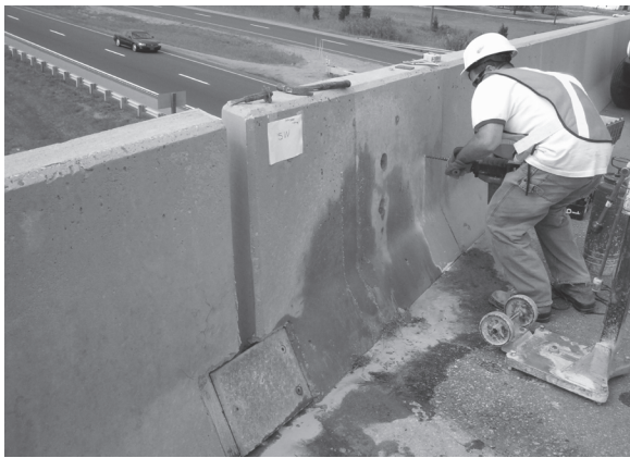
Figure 3 – Barrier wall of Chatham Bridge.
