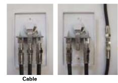
If your outside TV receptacle is wired for **satellite**, you'll need to locate where that receptacle leads, and connect that directly to your satellite receiver. If the outside TV receptacle is wired for **cable**, the wiring will have to be modified for use with satellite. The coaxial cable cannot run through any other devices or switches **BEFORE** the satellite receiver.
