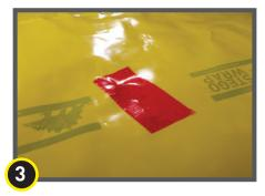
Center Stego Tape over small hole or slice in Stego Wrap.
