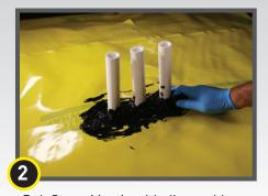
Dab Stego Mastic with disposable glove, paint brush, or similar, making sure entire void space is sealed.
