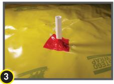
If Stego Wrap is close to pipe and void space is minimized then seal around pipe penetration with Stego Tape and/or Stego Mastic.
