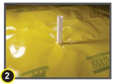
Pull material over and flatten. Clean area of adhesion where Stego Tape will be applied.
