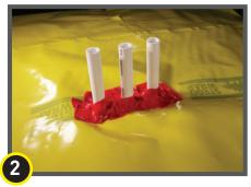
Seal any void space around each pipe using Stego Tape.
