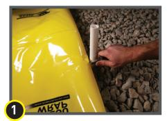
Install Stego Wrap around pipe penetrations by slitting/cutting material as needed. Try to minimize the void space created.
