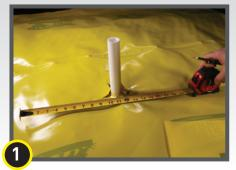
Cut a detail patch to a size and shape that creates a 6" overlap on all edges around the void space at the base of the pipe.
