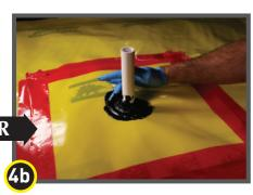
Seal around the base of the pipe with Stego Mastic. Note: apply using disposable glove, paint brush, or similar.
