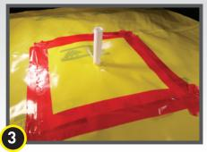
Seal all sides of the pipe boot with Stego Tape.
