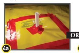
Seal around the base of the pipe using Stego Tape. **OR...**
