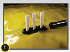
Seal any void space around each pipe penetration with Stego Mastic.
