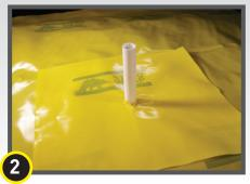
Cut an "X" the size of the pipe diameter in the center of the pipe boot and slide tightly over pipe.
