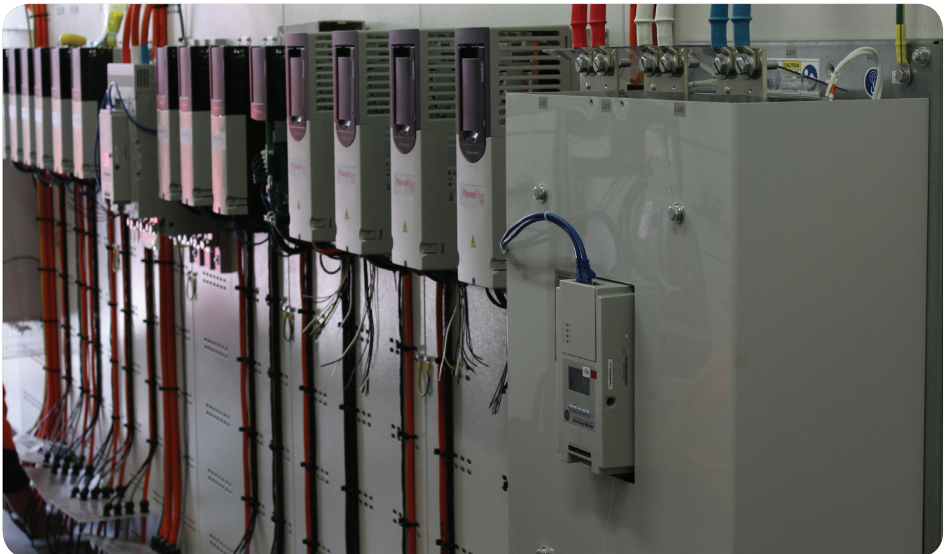
More than 75 variable speed drives were required due to the size of the plant
