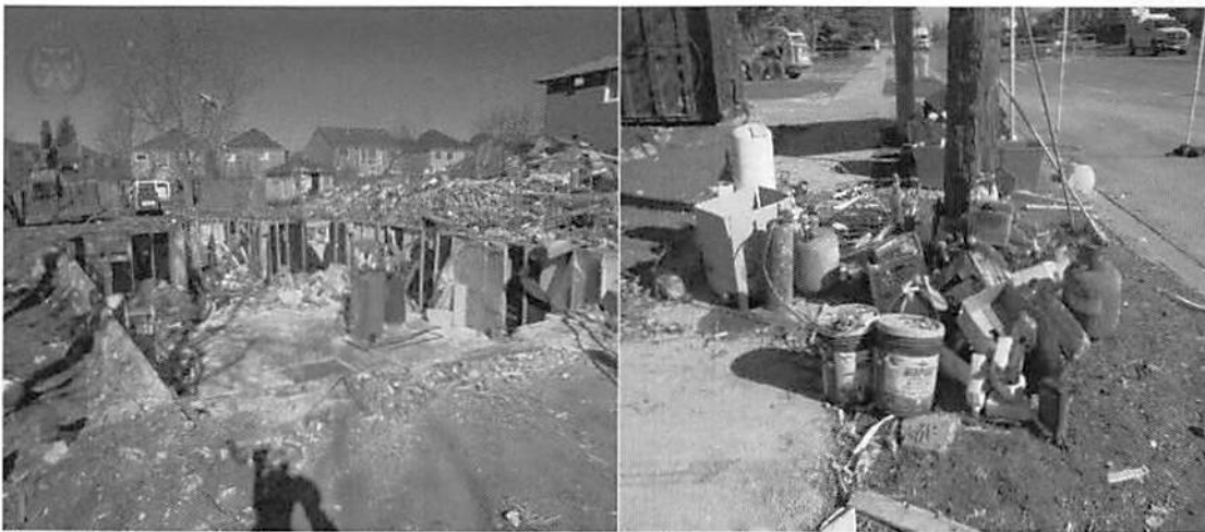
Figure 9- Excavated basement interior and recovered items.
