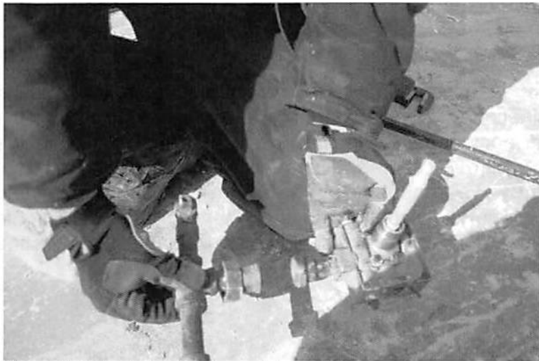
Figure 8 - Detached natural gas piping union.
