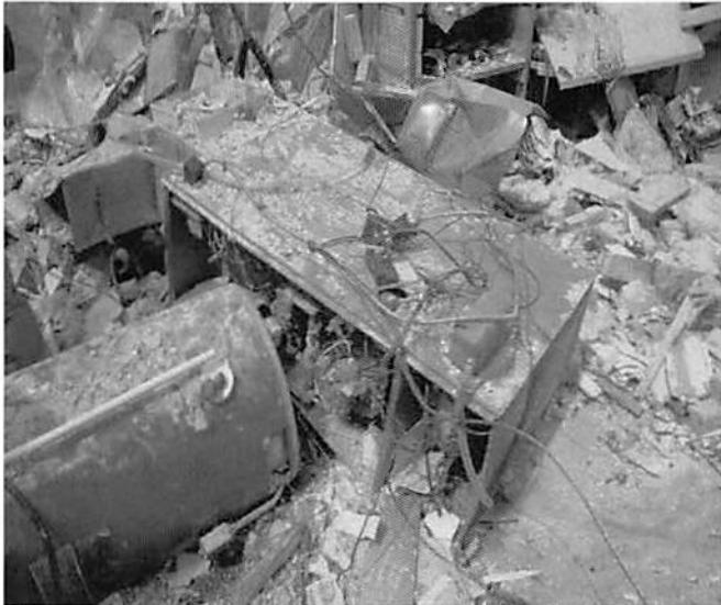
Figure 6- Furnace and Hot water heater in situ.
