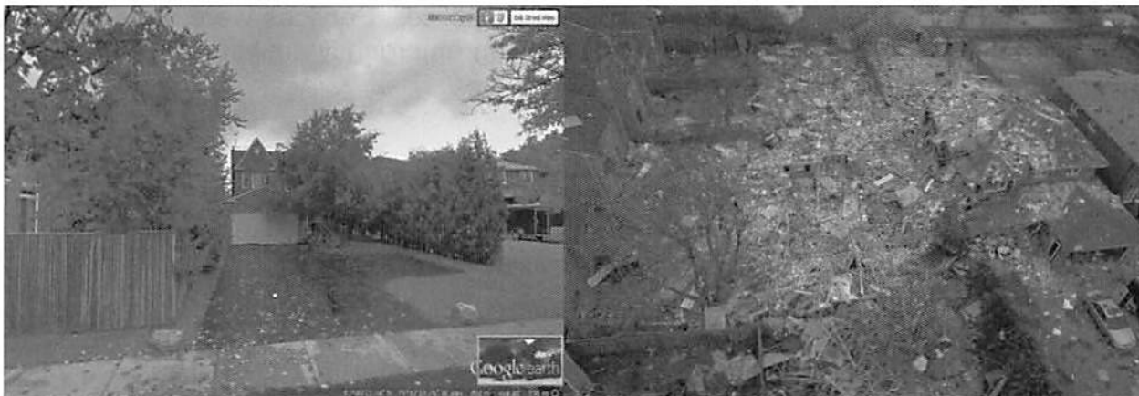
Figure 1 – Pre-explosion and post-explosion exterior of residence
