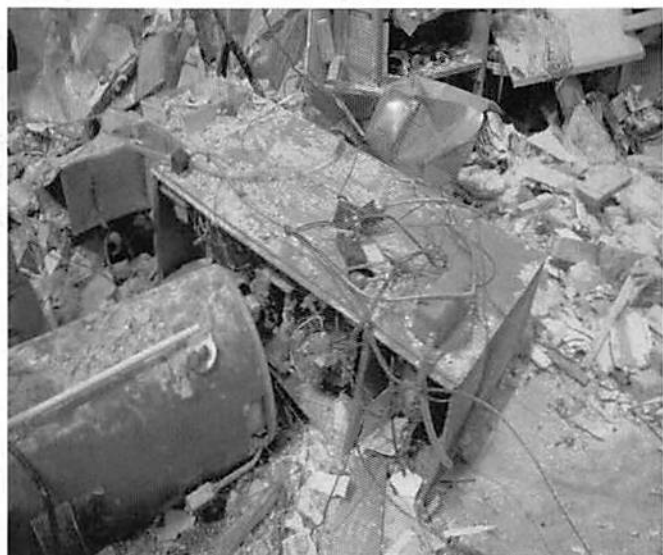
Figure 6- Furnace and Hot water heater in situ.
