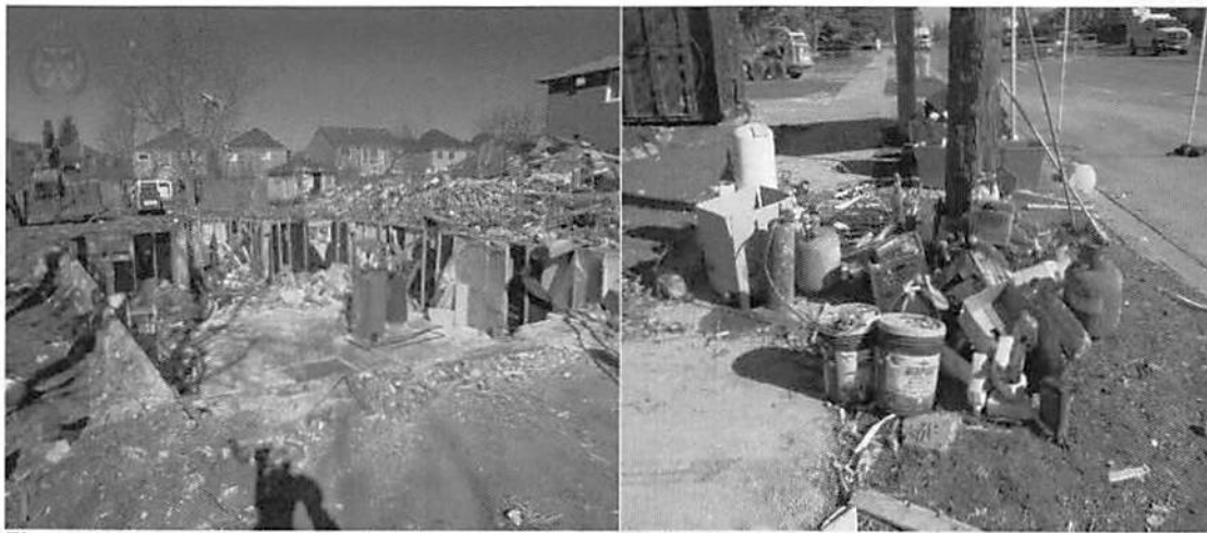
Figure 9- Excavated basement interior and recovered items.
