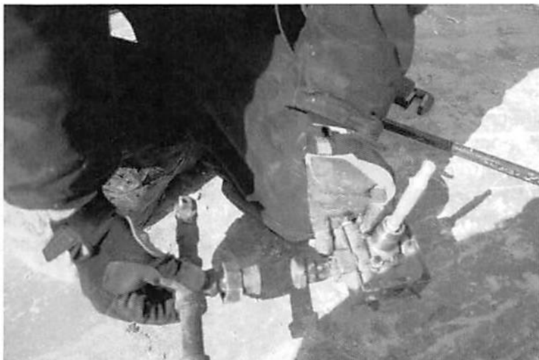
Figure 8 - Detached natural gas piping union.
