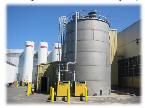
**The Problem:** The Nation's Largest Soft Drink and Juice Bottling Company was operating an MBR system that was not performing to maintain the flow rate required for effluent discharge. The Membrane System had rapid flux decline and the tubular membranes failed after 6 months resulting in the company bypassing the membrane system altogether.
