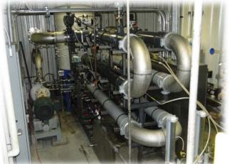
**The Problem:** The Nation's Largest Soft Drink and Juice Bottling Company was operating an MBR system that was not performing to maintain the flow rate required for effluent discharge. The Membrane System had rapid flux decline and the tubular membranes failed after 6 months resulting in the company bypassing the membrane system altogether.
