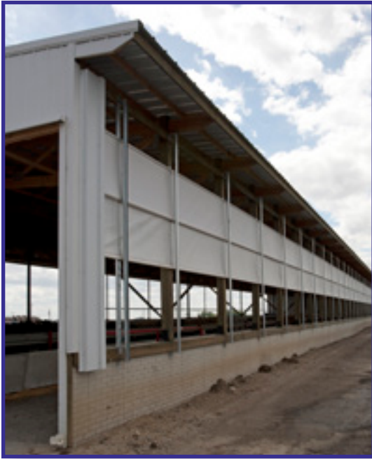
Curtain application on a Summit Livestock Facilities monoslope beef barn.
