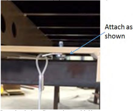
4.7.2 Use a 9/16" wrench and a 6mm allen wrench to attach ladder.
