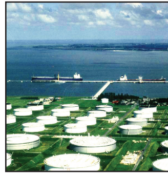
Bulk Petroleum Terminal Retrofit
