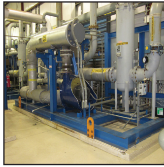
Site Investigation Former Glass Manufacturing Facility
