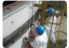
Plate Bonding Repair of Thin & Through-Wall Damage to Metal Structures Fast Application
