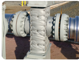
Insulation Blankets Removable for Maintenance and Inspection of Flanges, Valves, Pump Boxes, etc.
