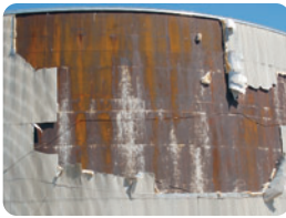
Insulation Repairs Vertical, Horizontal & Foam We Can Fix It Start-to-Finish Service
