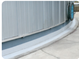
CUI Repairs Hidden CUI Threatens Shutdowns and Product Loss, We Can Find It, We Can Fix It!
