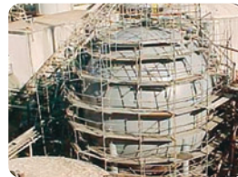
Scaffolding Services OSHA Compliant ♦ Tanks Vessels ♦ Painting ♦ HVAC We Solve Difficult Applications
