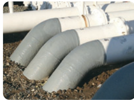
Soil Line Pipe Corrosion Repair of Thin or Through-Wall Damaged Pipe to ISO, ASME & US DOT Code Standards
