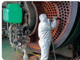
Boiler Services Installation ♦ Repair ♦ Re-Tubing Casing Repairs Handhole/Manways
