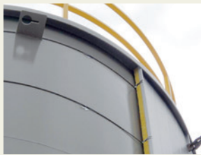
Clips anchor to cables.
