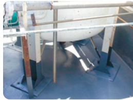
Vessel Support Repairs Repair and Protection of Metal & Concrete Supports for Pipes & Vessels
