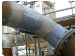
Pipe Leak Repairs Fast Solutions to Repair and Strengthen Pipes Damaged by Corrosion or Abrasion
