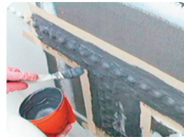
Joint & Seam Repairs Prolong Asset Life ♦ Save Money Emergency Leak Sealing Using External Bonding
