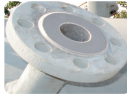
Flange Face Repairs Fast Repair and Protection of Damaged Flange Faces at a Fraction of Replacement Cost
