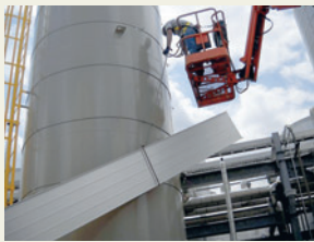
Panels are positioned.
