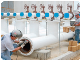
Mechanical Services Pipe Fabrication ♦ Support Repair ASME Certified Welders Plumbers ♦ Riggers ♦ Operators
