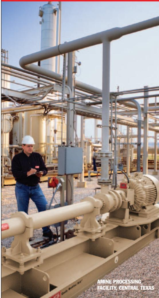
Our multi-stage centrifugal Surface Pumping System (SPS) provides a versatile, low-maintenance alternative to many split-case centrifugal, positive-displacement and vertical-turbine pump applications. The SPS is a cost-effective solution for petroleum, mining, processing, water and other industries that require high-pressure movement of fluids. Proven benefits include:
