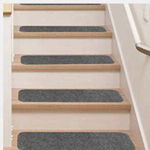
Apply non-skid treads to each step.
