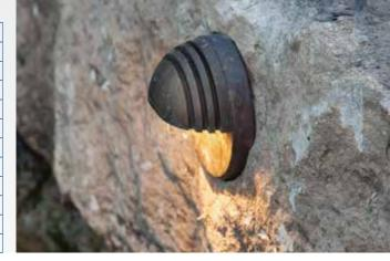
Above, Right: The lighting team used an angle grinder to create a flat surface for mounting the wall fixtures. A hammer drill penetrated the limestone slabs, creating holes as deep as three feet so wires could be threaded through to connections in the back of the wall.
