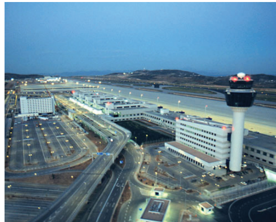
Athens International Airport
