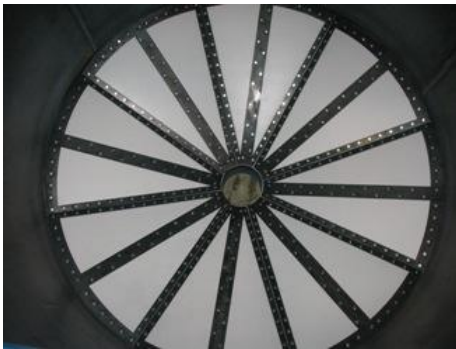
AERATED FLAT BOTTOM HOPPER (INSIDE VIEW)
