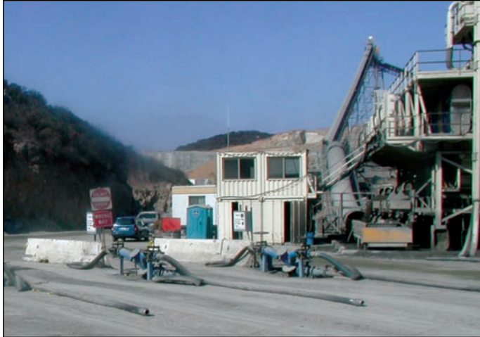
Turbo-Inductor installation with lines ready to connect to PD trailers.
