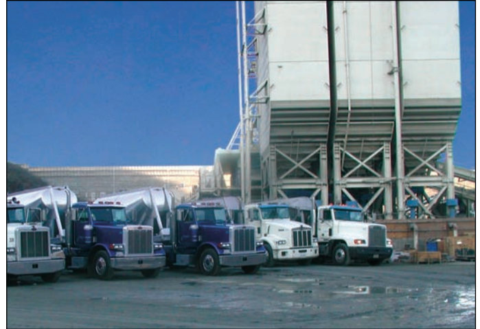
Trailers loaded with fly ash line up to unload their cargoes into bulk storage silos.
