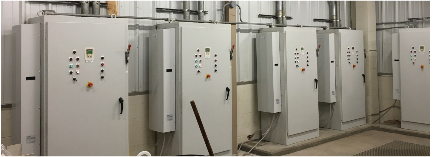
Pfannenber air-to-water heat exchangers in the pump control room of a wastewater treatment plant.
