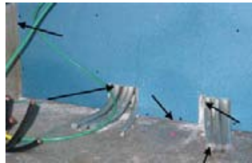
Air leakage in an underfloor air-distribution system [Stum 2008]
