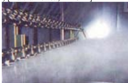
Active humidification downstream of a condensing cooling coil at cleanroom facility [Sellers no date]
