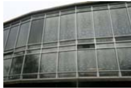
Failed window film treatment.
