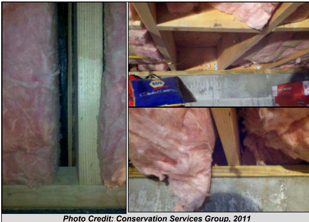
Figure I- 8: Examples of Grade III Insulation Installation
