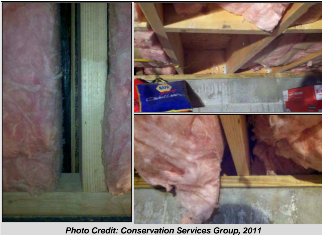
Figure 4- 4: Examples of Grade III (poor quality) Insulation
