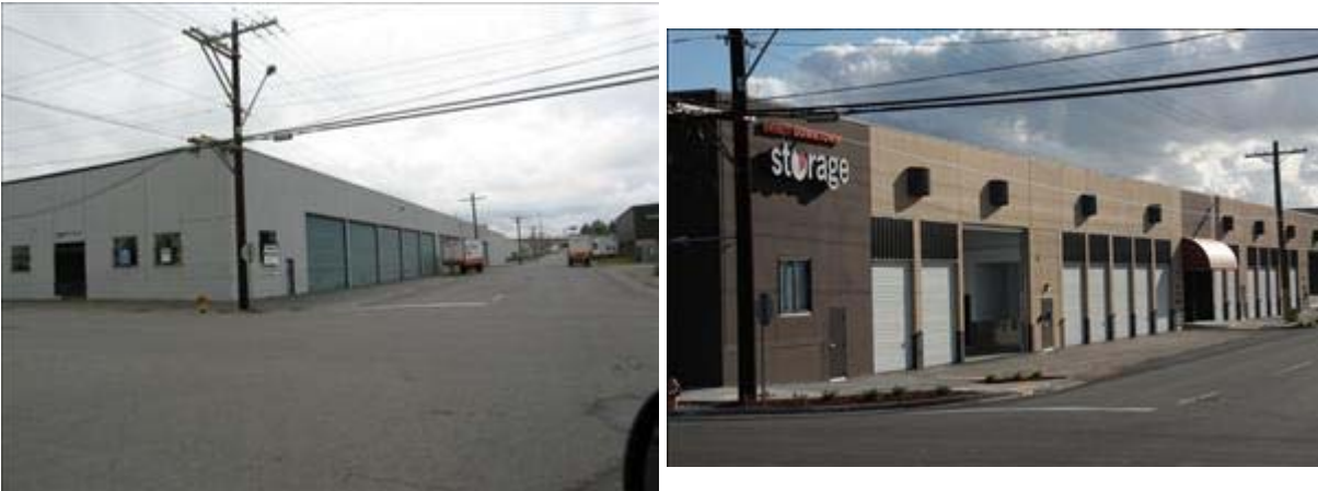
Everett Downtown Storage in Everett, Wash., before conversion (left) and after (right).
