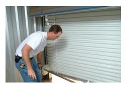
**9.** Line the hole on the brackets up with the holes left in the jamb. Secure the Janus bracket to the wall using appropriate fasteners supplied. Repeat this step on the other bracket.
