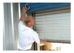
6. Using the screw gun, remove the teks screws attaching the curtain to the axle assembly.
