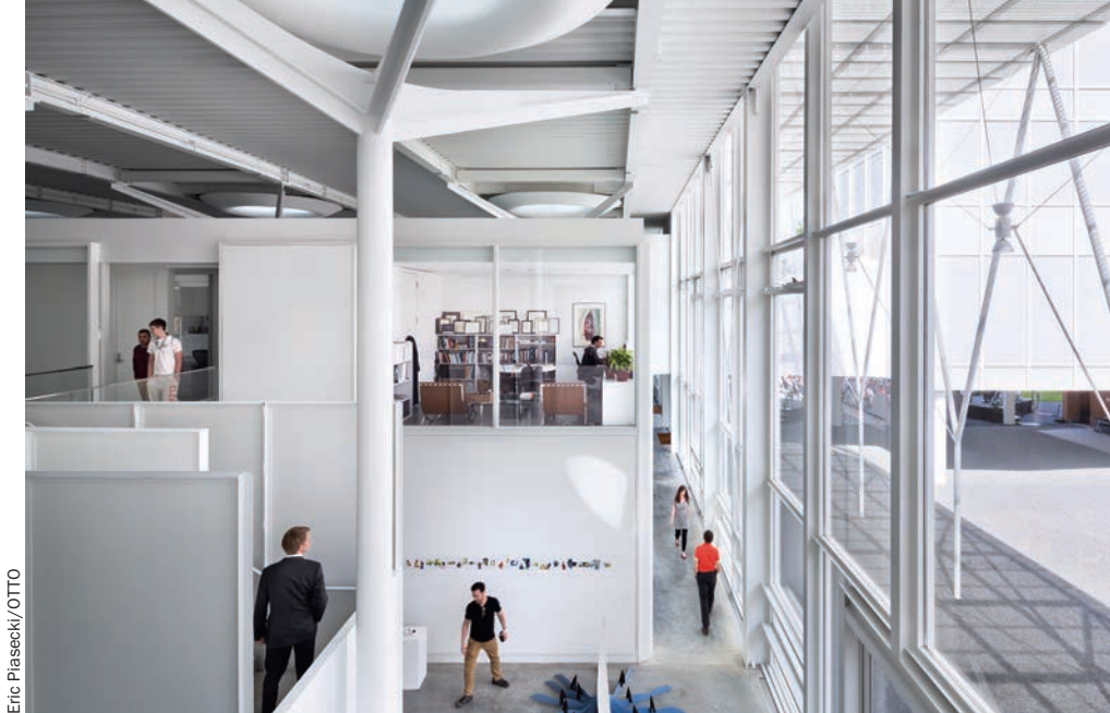
Detail of the perforated roof/ceiling of the north porch featuring one of the tethered light fixtures.
