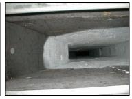
Another option to cleaning and coating is to replace the damaged/degraded mechanical insulation with closed cell insulation. You remove the existing insulation; measure and cut the appropriate size close cell insulation; then glue and rivet the close cell insulation in place; seal all exposed edges and butt joints. The benefits of relining with closed cell insulation include:
