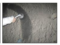
Normal cleaning methods include contact vacuuming or cleaning with a powered brushing system/robotic system with a nylon brush and then air washing. This removes the dirt/contamination from the surface of the insulation but does not remove the dirt/contaminating form the interior of the fiberglass insulation. To keep this dirt/contamination in the interior of the fiberglass insulation from becoming a future problem you can coat the mechanical insulation. The benefits of coating include:
