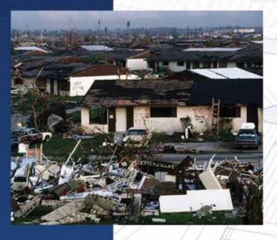
It is now well known that flying debris will break normal windows, which can cause a sudden internal pressurization within your home. This is a common cause for most roof failures. By having impact-resistant glass, you significantly improve the homes structural integrity and can avoid any potential "breach of the home's envelope." Our systems provide maximized resistance and certified protection.
