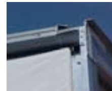
Rear header upper rain gutter
