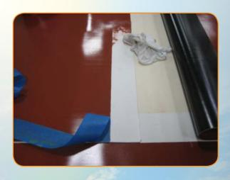
Do not spill the M.E.K. onto exposed FiberTite Brite. It will cause damage to the top coating.
