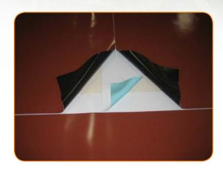
For the concealed butt seam, use a minimum 4-inch wide piece of FiberTite Brite base membrane without the topfinish. Align the piece centered directly below the ends of the membrane. A 6-foot straight edge comes in handy to make even and straight cuts. Weld the tongue of the base membrane then weld down the ends to the base.
