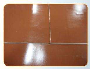
To complete standard end laps, the Kynar top-finish will need to be removed. Overlap the roll ends by about 3 inches.
