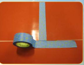
Fold back the lap. Using a clean, white, cotton rag, remove the Kynar with a liberal application of M.E.K.
