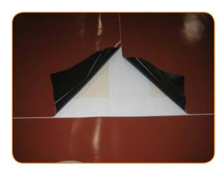
Masking and general lap assemblies require 90-degree corners; so do not round the membrane corners.
