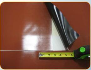
Lap the roll ends approximately 3 inches and mask the lap area using FiberTite Scotch Blue tape. Keep laps and edges straight and square. This will help reduce the amount of general touch-up required upon completion.
