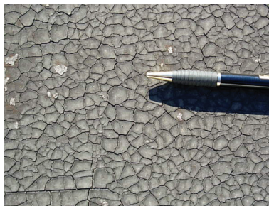
(Top) UV light has caused alligatoring on this bituminous roof.
