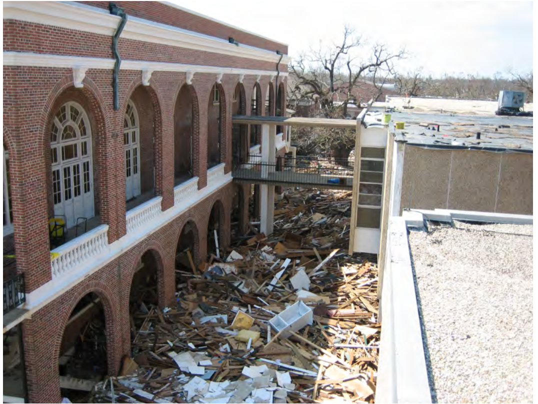
Here too the school suffered complete destruction of the lower level from the storm surge with apparent flooding on the second floor.
