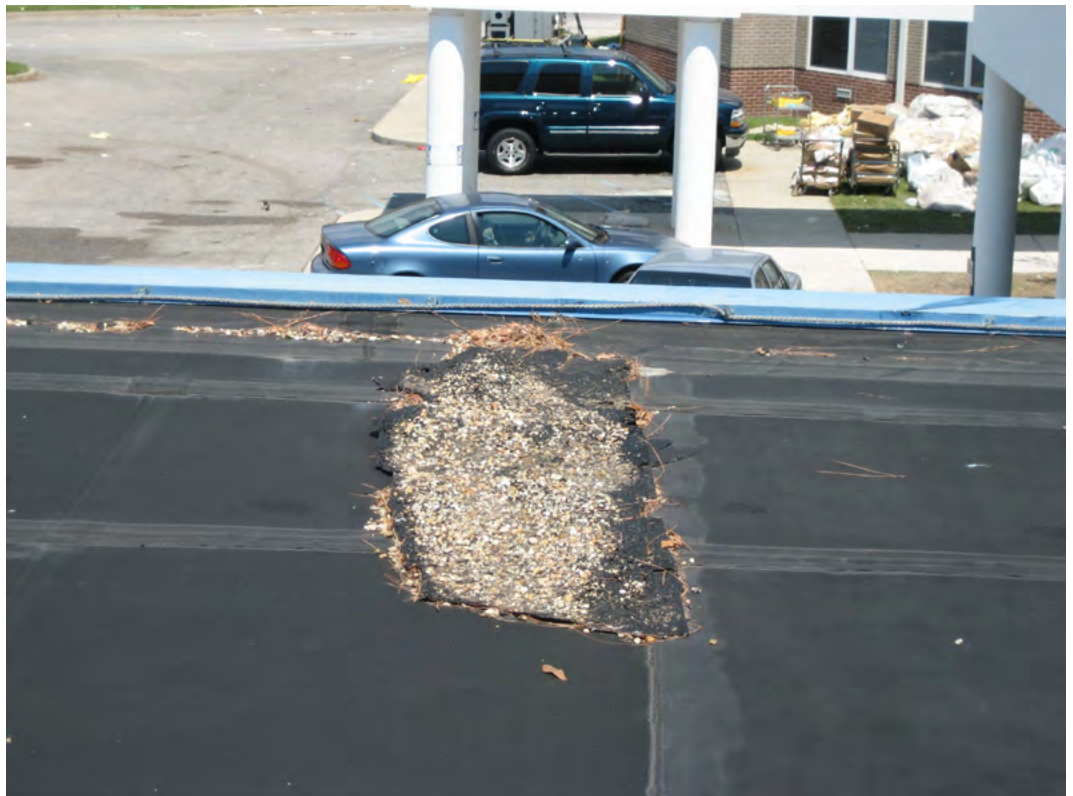
Debris from a built up roof system with no apparent source.
