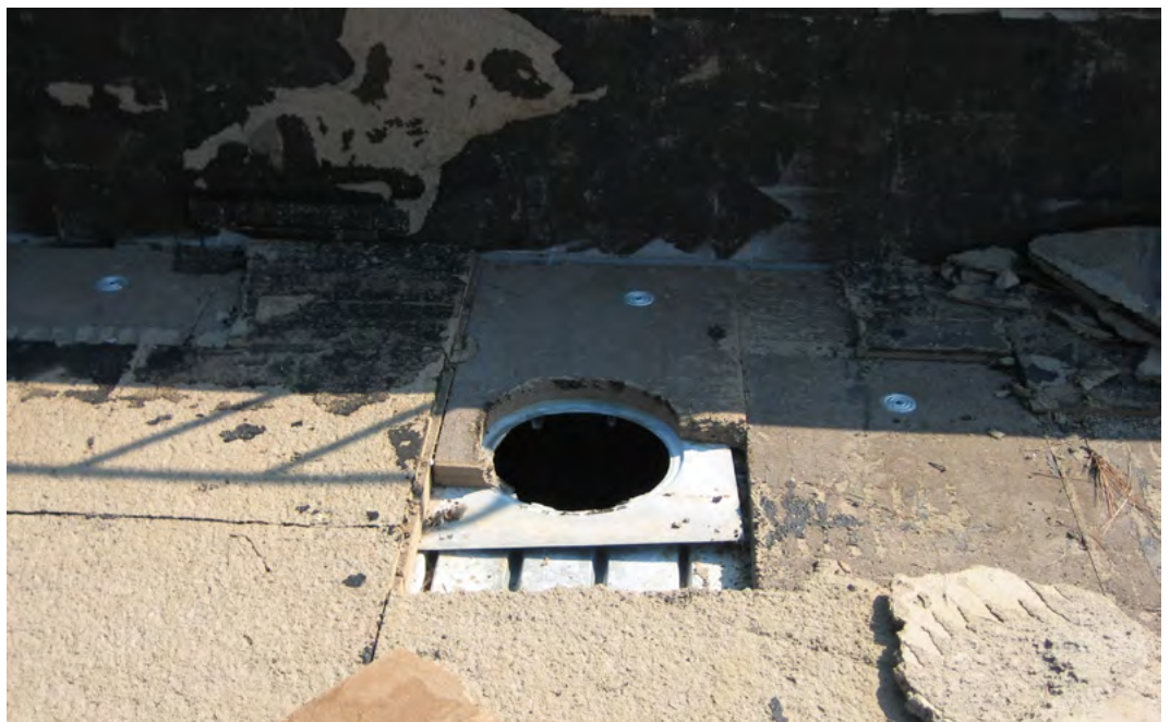
This was the roof drain. It was located directly above the rolling freight door. Note the “fasteners” in the base layer of perlite.
