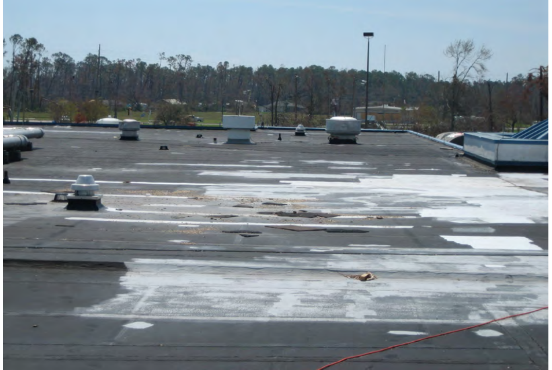
Hospital; Mechanically Fastened EPDM.
