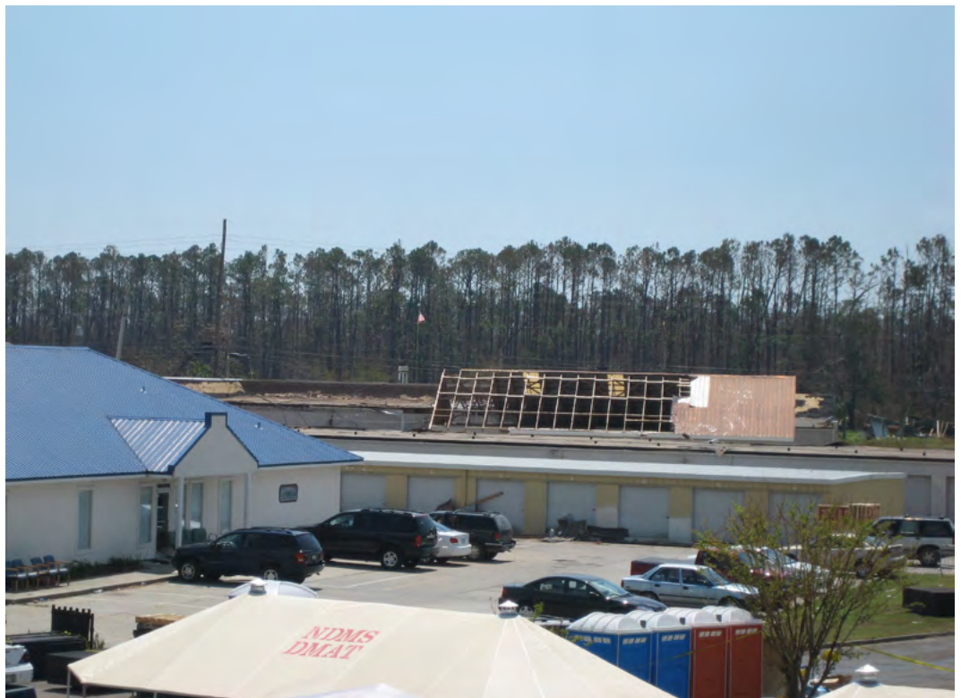
Small Strip Center off to the south east that was the source of the debris on the hospital roof.
