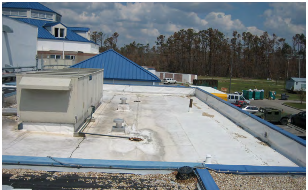
Hospital; Mechanically fastened vinyl roof system.
