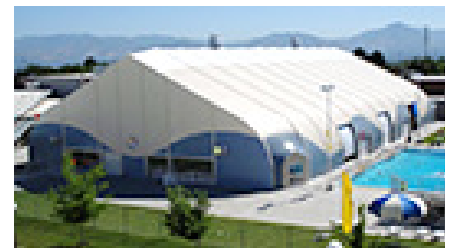
Shown is a pre-engineered architectural structure that uses fabric with a protective top finish.
