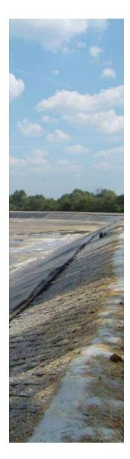
The City of Franklin, located just outside of Nashville, Tennessee, selected Seaman Corporation's potable water grade XR geomembrane fabrics to line its 35-acre raw water storage reservoir. The raw water reservoir is the sole source of water for the existing 2.0 mgd water treatment facility located on an adjacent site.
