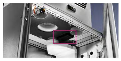
These use an efficient PTC heating cartridge with automatic adjustment of thermal output depending on the amount of condensation. Approx. 120 ml of condensate can be evaporated per hour. This ensures complete removal of condensate.
