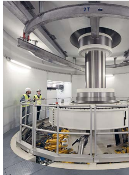
Figure 14: Frades II commissioning
