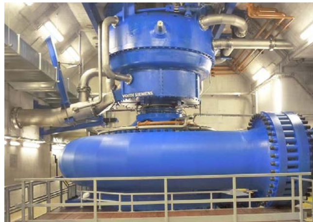
Figure 10: Cross-section and photo of the Kops II hydraulic torque converter
