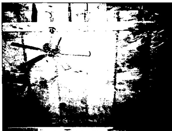
Black mold can be a problem in homes lacking an air barrier. Here, black mold grows in three-year-old insulation installed in a cathedral style ceiling.
