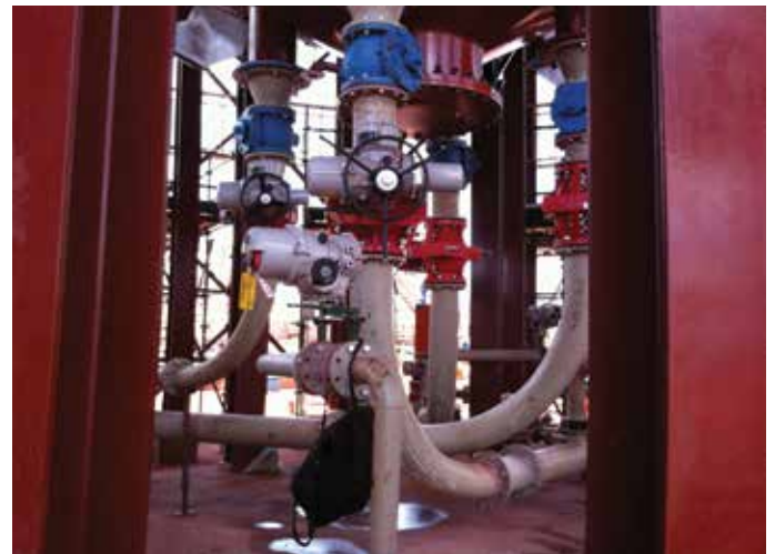
Underflow Control System
