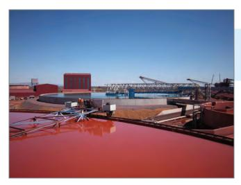
For high-tonnage / high-torque applications, a WesTech Titan<sup>TM</sup> traction thickener can be used as an ideal, economical alternative to conventional center-driven, high-rate thickeners.
