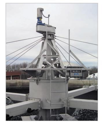
The average U.S. trickling filter distributor should be slowed to 5-10 percent of its current rotational rate.
