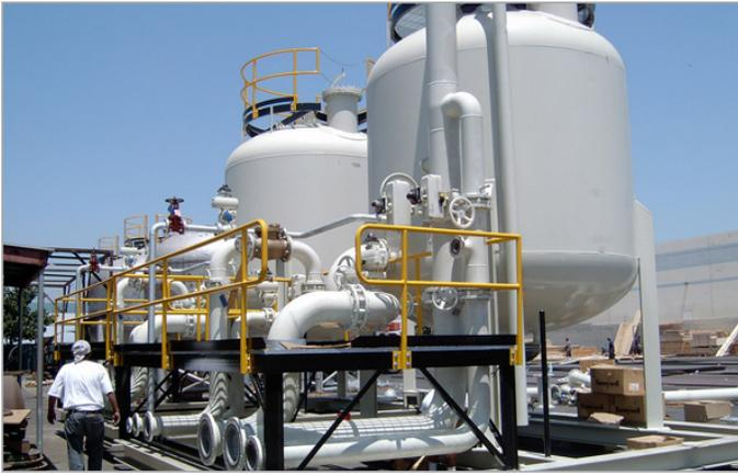
WesTech **Pressure Filtration Systems** are designed for industrial water treatment where the removal of suspended solids such as particulates, iron, manganese, free oils, mill scale, and other precipitates in ground or surface water is required. Pressure filters are commonly placed after WesTech clarification equipment. When used as pretreatment equipment, these filters will prolong the life and efficiency of granular activated carbon, ion exchange, and membrane systems.
