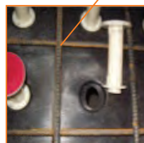
Install Pan-Form Rebar and Twist-Lock Nozzle Inserts
