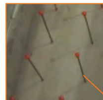
Epoxy Rebar into Basin Floor
