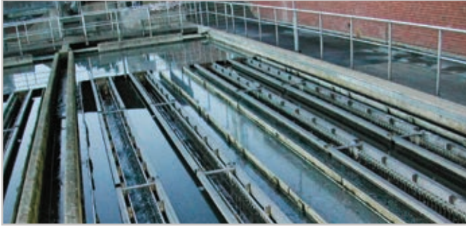
SuperSettler Tertiary Treatment at Rosenholms WWTP, Sweden in operation since 1977
