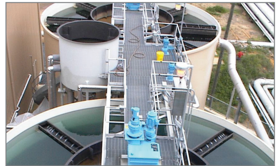
Industrial Surface Water Clarification
