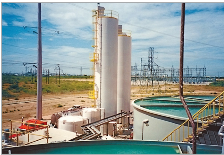
Lime / Soda Ash Storage
