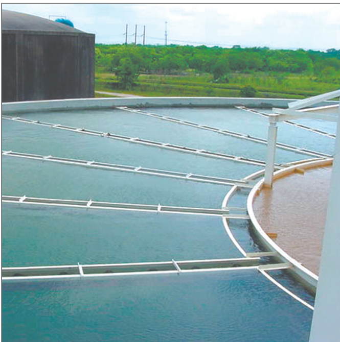
Surface Water Clarification
