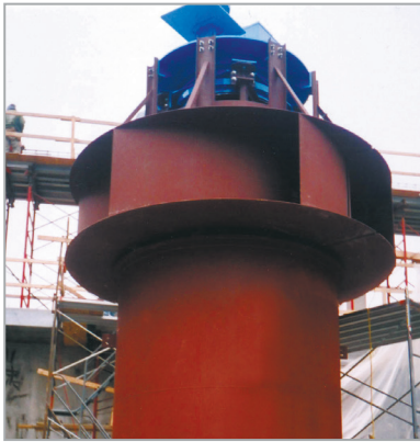
Centrifugal Impeller Pump and Draft Tube
