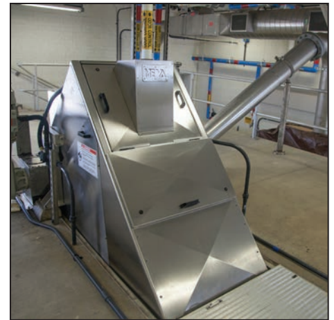
CleanFlo™ Monoscreen® installation
